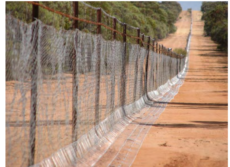
Upgraded State Barrier Fence with lap wire.
