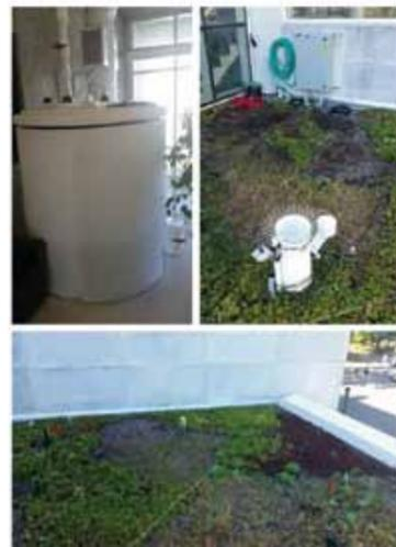
Figure 8. The CMAC green roof at Villanova University (bottom); indoor cistern collecting runoff from additional, non-green roof to be used for irrigation of green roof (top left); control panel and weather station (top right)
