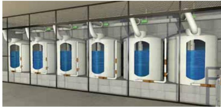
Figure 4. Six, 1,000-gallon (3,790-liter) cisterns in the basement of EPA headquarters in Washington, D.C., collect runoff from the building roof to be used for on-site irrigation. Adaptive control of the cisterns has reduced wet weather flow to the combined sewer by 80 percent.
