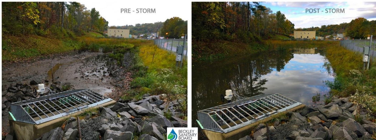
Completed iPond, detaining runoff from the Ewart Ave subwatershed, thereby preventing flooding downstream at the convergence of watersheds.
