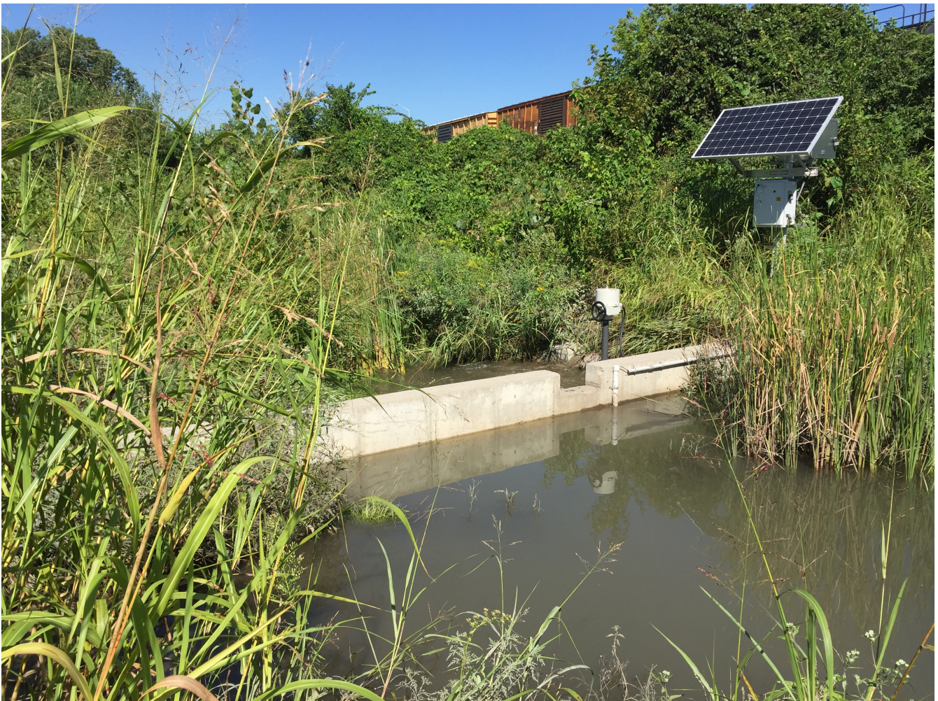
Gardner Avenue Detention Facility
