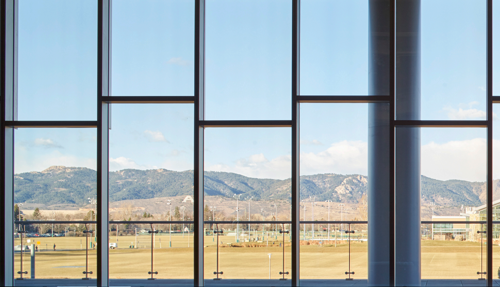
CSU Lory Student Center Fort Collins, CO Architect: Perkins + Will
